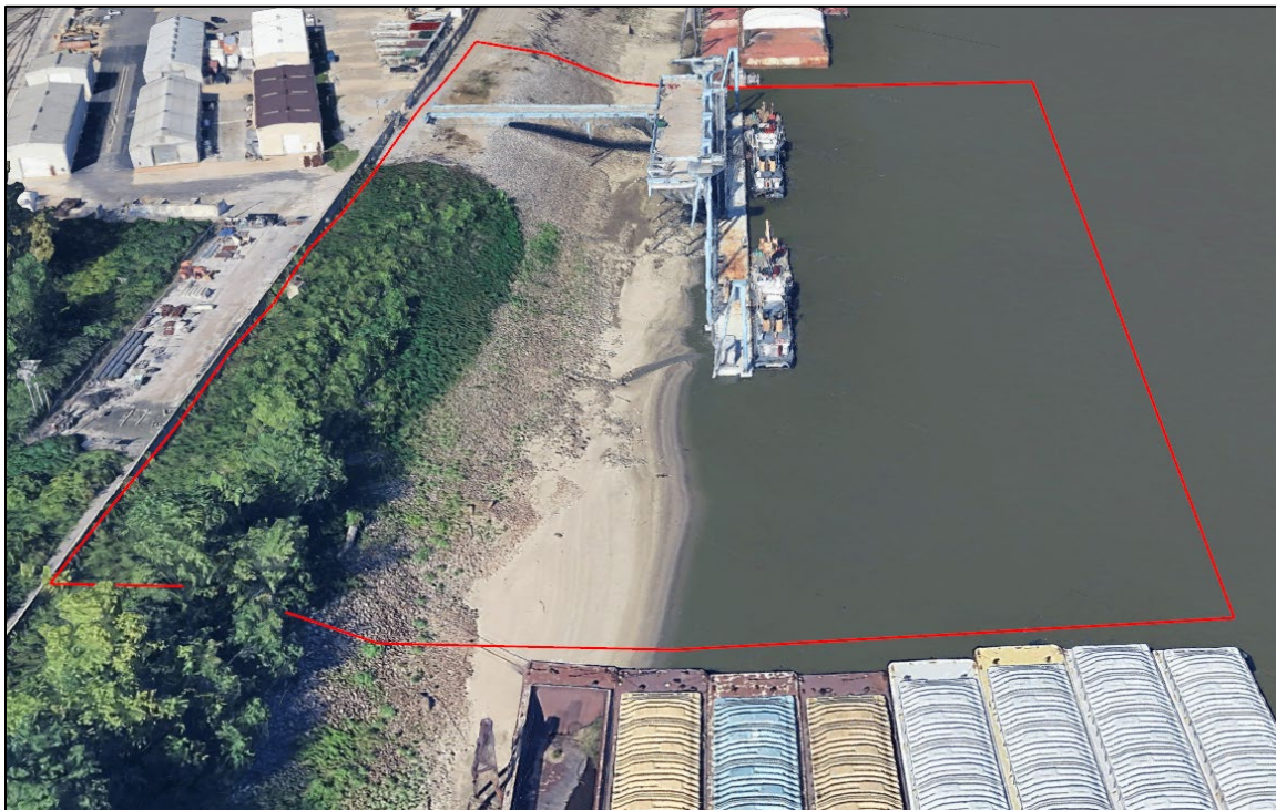
Figure 3-2: 3D images of the site (facing upstream/northeast, Google Earth August 2023) showing bank slope and the existing dock, floating docks, and moored cutters at the facility. Fleeted barges are visible in the foreground.
