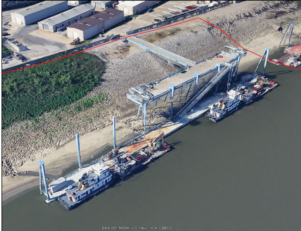
Figure 3-1: 3D image of the site (facing west bank, Google Earth August 2023) showing existing floating docks, wharf, and rip rap.
